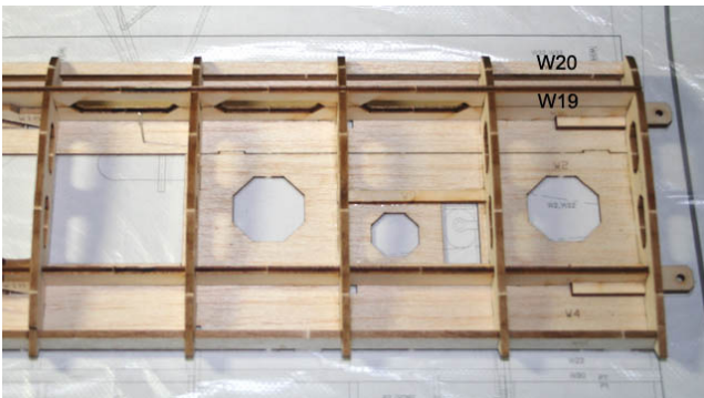
5. Assemble and glue plywood upper spar(W19) and sub leading edge(W20) with thick CA.
